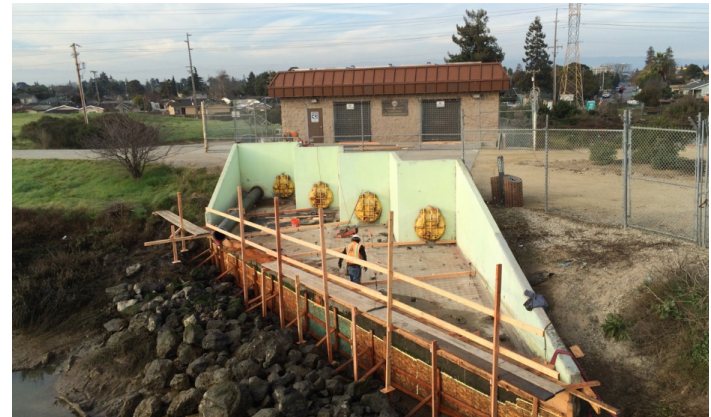
Pump Repair Project
