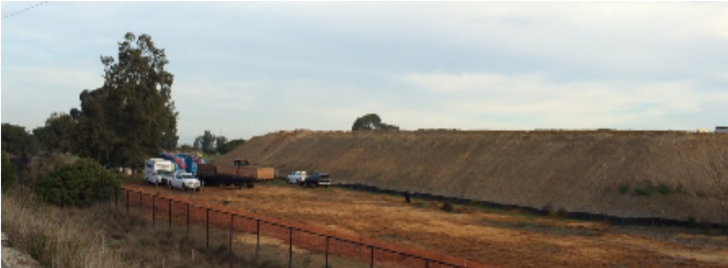
Levee Reconstruction and Recertification
